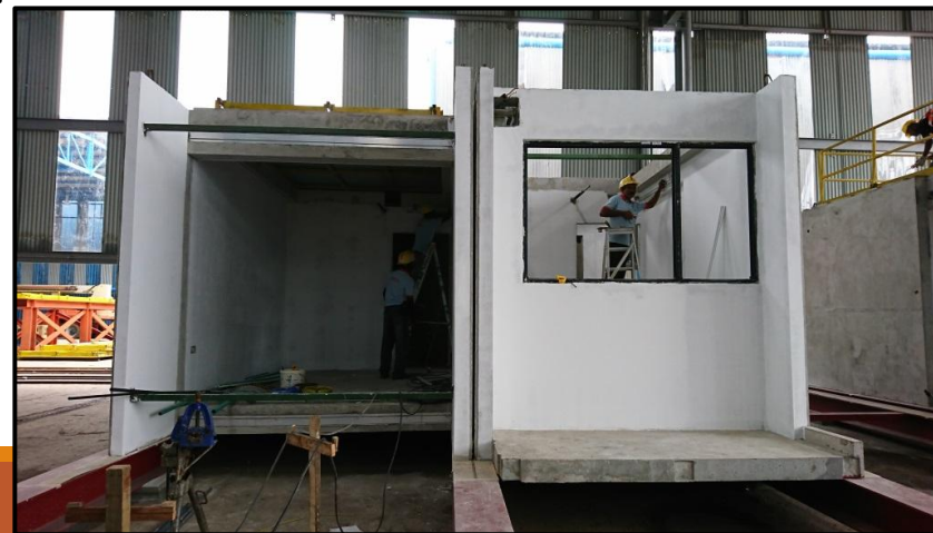
30% Architectural Fit Out at Factory (offsite)
