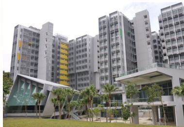
NTU North Hill Hostel (PPVC)
