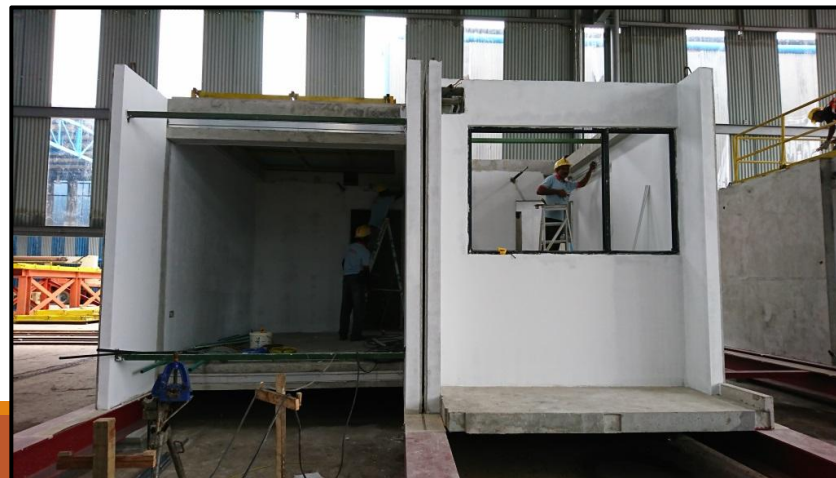
Architectural Fit Out at Factory (offsite)
