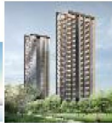
40-Storey Clement Canopy Condominium (PPVC)
