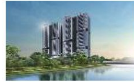
36-Storey Parc Riviera Condominium (PPVC)
