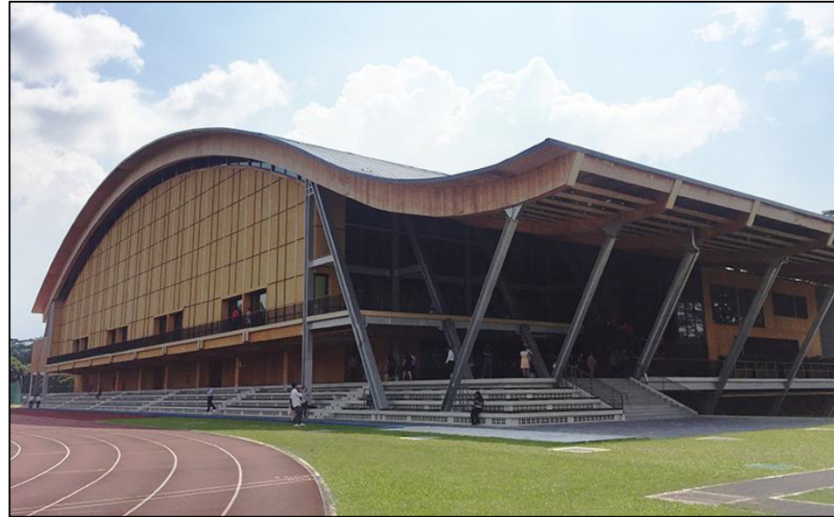
Mass Engineered Timber (MET)
