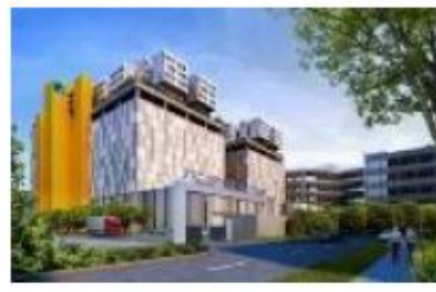
9-Storey Dormitory at JTC Space @ Tuas (PPVC)
